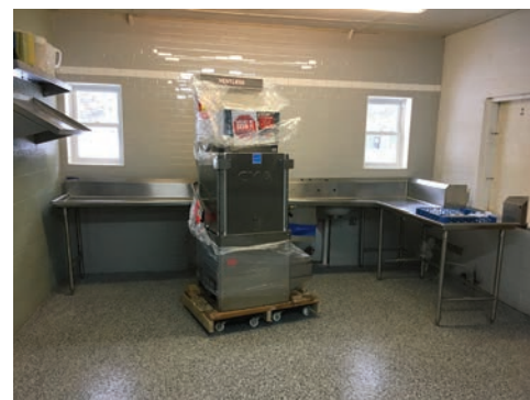
2017 NEW epoxy floor installed in kitchen
